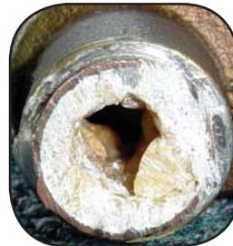
*When scale build-up is this bad, you must replace piping before installation of a water softener to prevent pipes from corrosion and possible leakage.*
